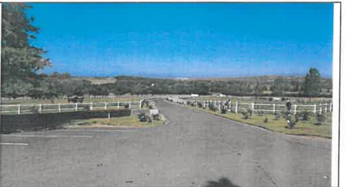
Internal access road
