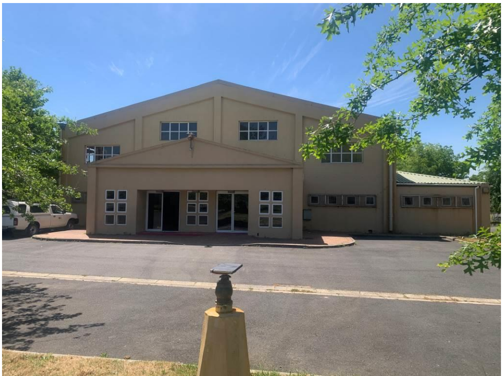
Figure 2: Front of the Millennium Hall
