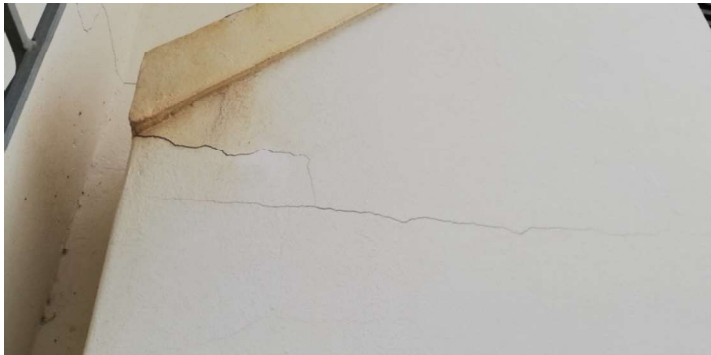
Figure 9: Cracked wall
