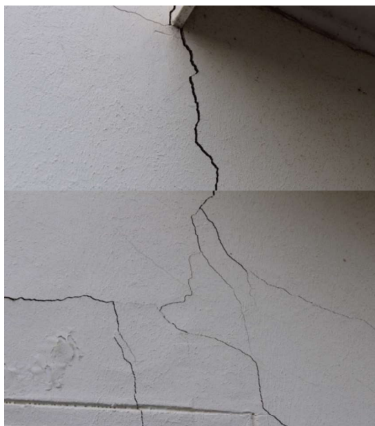
Figure 13: Separation crack
