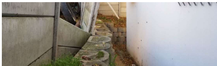
Figure 51: Out of plan movement of Terraforce wall
