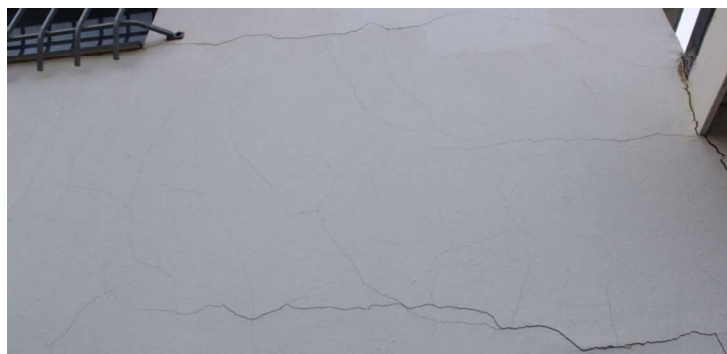
Figure 12: Horizontal cracks
