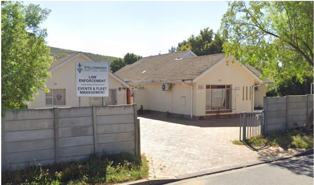
Figure 3: Front of building. New entrance gate to be installed.
