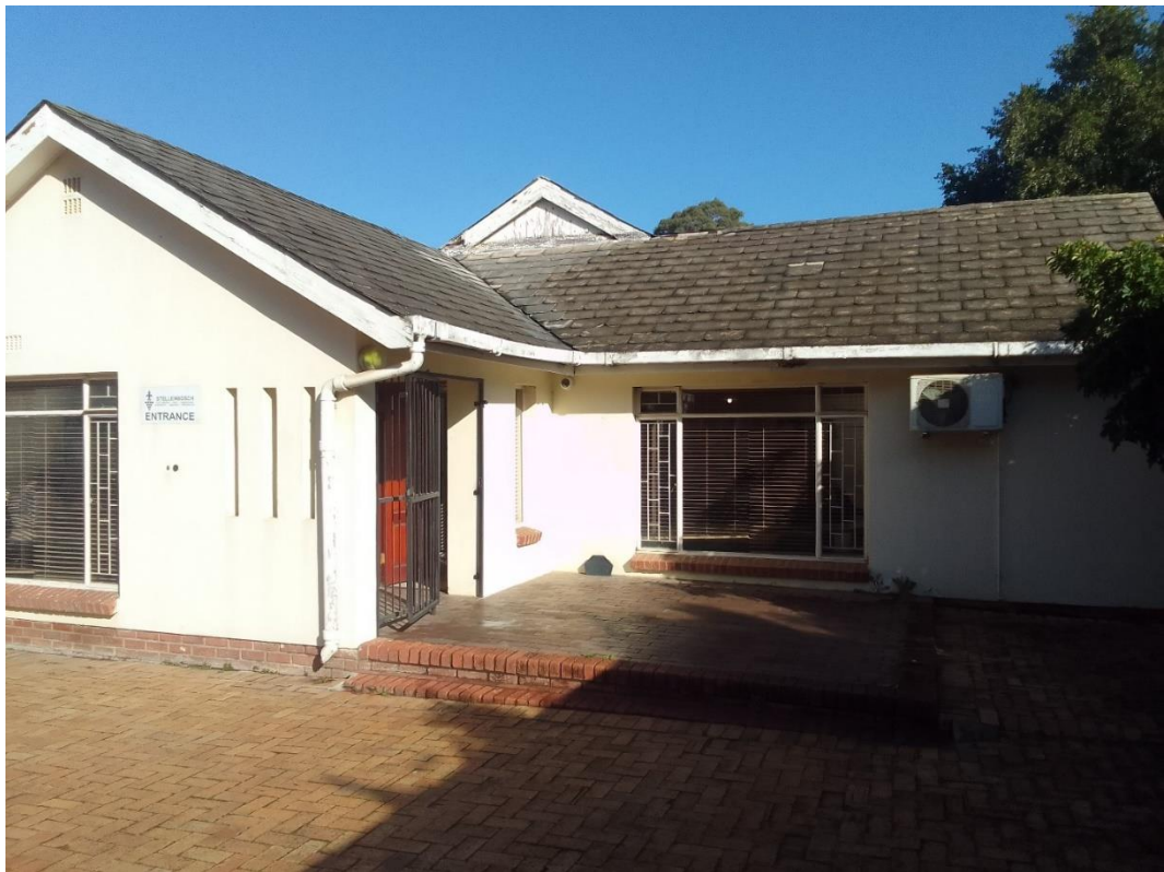
Figure 6: Photo indicating new position of entrance and construction of ramp.
