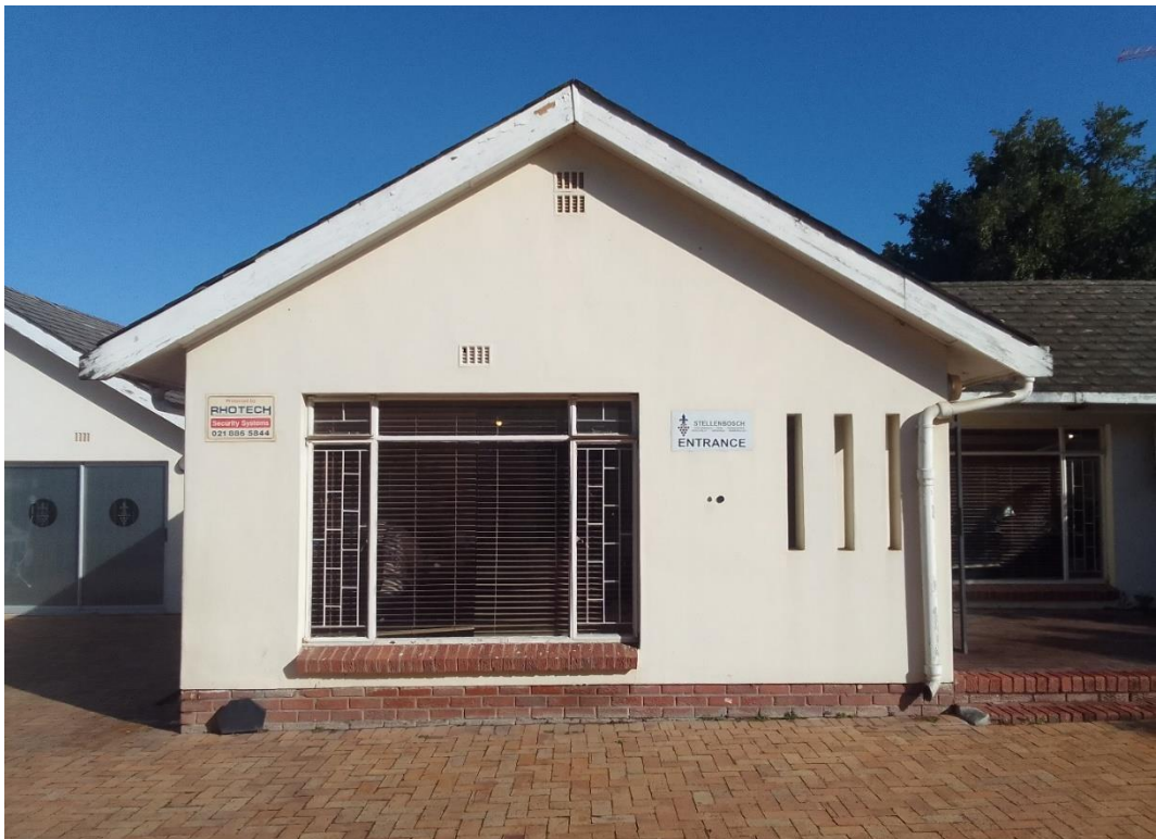
Figure 4: Photo indicating position of new extension.
