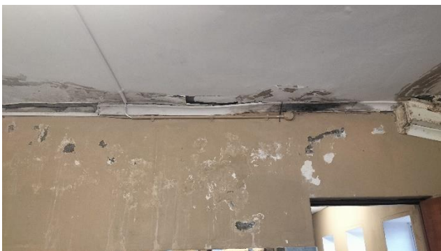
Photo 11: Water damage to internal wall. Wall directly below bridge connected to building.
