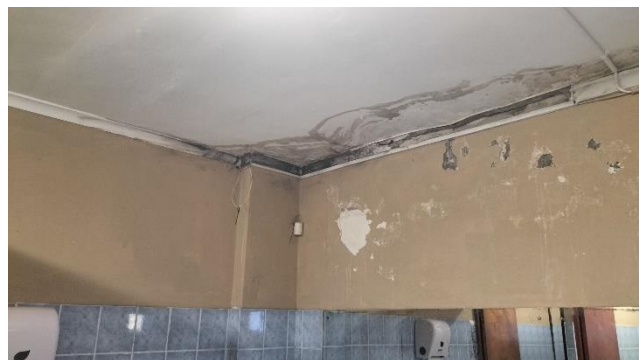
Photo 11: Water damage to internal wall. Wall directly below bridge connected to building.
