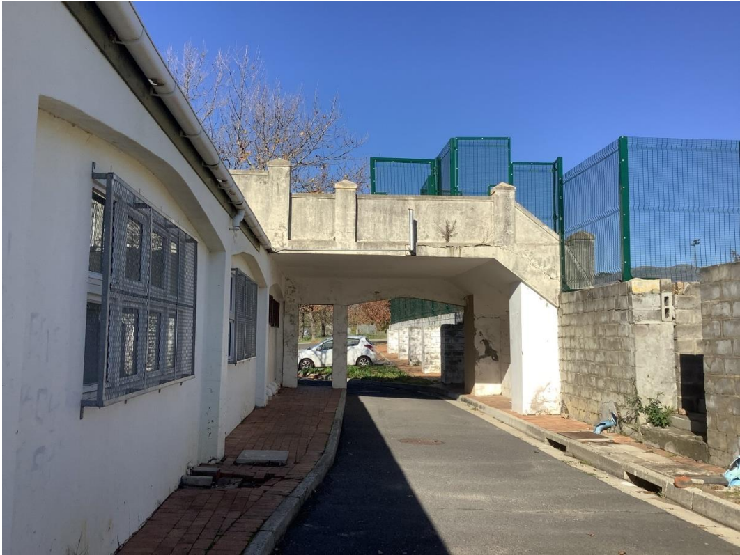
Figure 8: Photo of bridge from gym (left) to netball courts (right).
