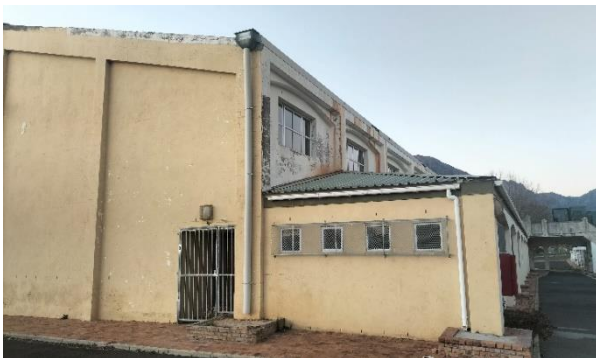
Photo 1a: Main gutter down North downpipe.
