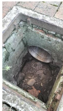
Photo 10: Catchpits without grid cover.
