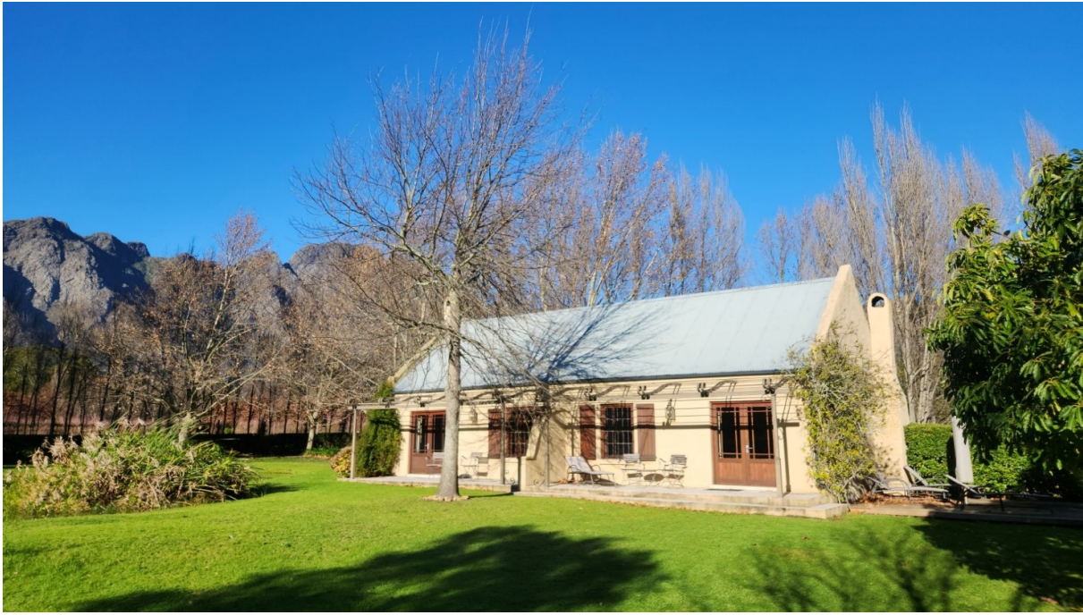
Figure 1: The original approved cottages on site.
