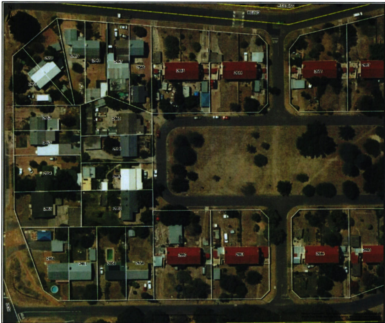
Figure 5: La Colline building development satellite image
