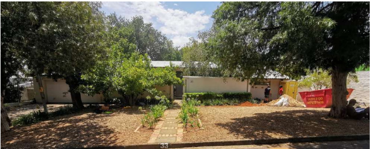
Figure 1: Street elevation of the dwelling on erf 1035, Stellenbosch.
