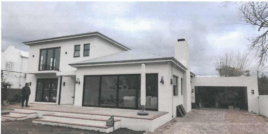
Figure 2: View of the residential dwelling on erf 870 currently being renovated. Note the addition of the first floor and the double garage.
