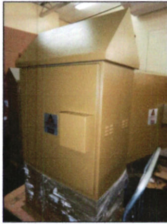
Figure 4 - Distribution/Metering Kiosk
