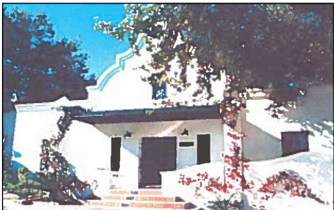
Figure 10: Existing Second Dwelling Unit
