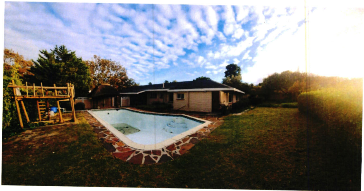
Figure 1: Street and rear elevation of the dwelling on erf 3567, Stellenbosch.
