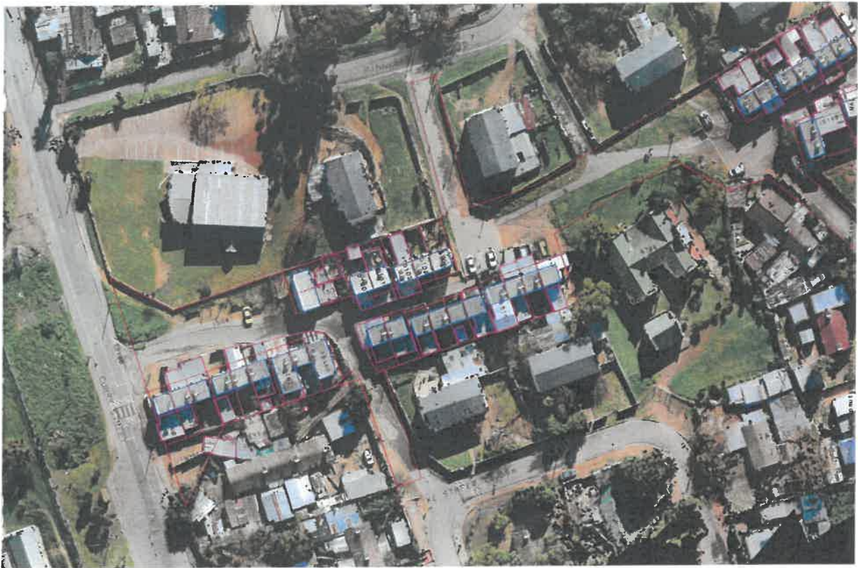
Figure 3.1: Drone survey of western portion of Remainder Erf 6846, with general plan superimposed to illustrate the extent and nature of encroachments (prepared by Middleton Geomatics, August 2023)
