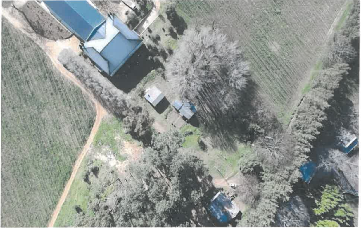
Aerial view of 3 existing cottages below the winery. A fairly damp low-lying area.
