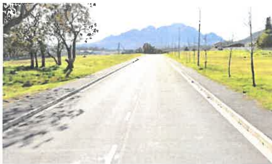
Figure 8: Fresno Street, Northbound
