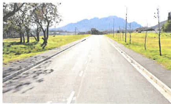
Figure 18: Existing NMT Facilities along Fresno Street, Northbound
