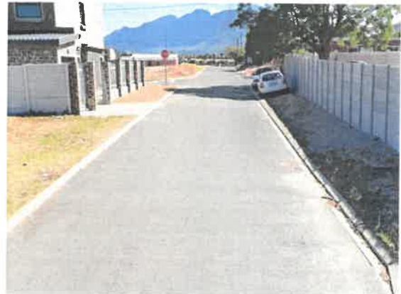
Figure 5: Blakemore Street, Northbound
