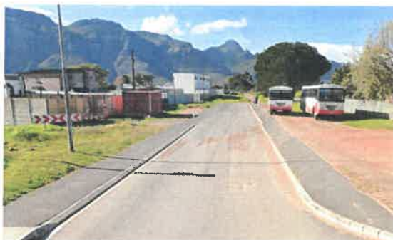
Figure 17: Existing NMT Facilities along School Road, Eastbound
