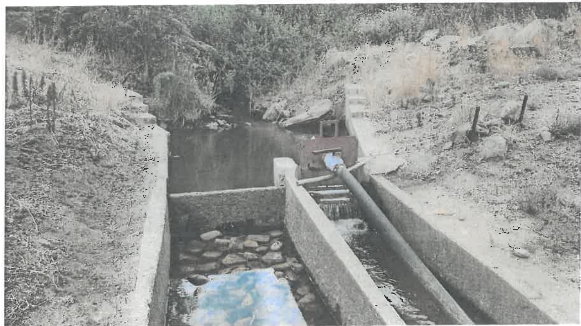
Image 6: Image shows a weir pond located at the upper north portion of the proposed site. Source: Antoinette de Beer
