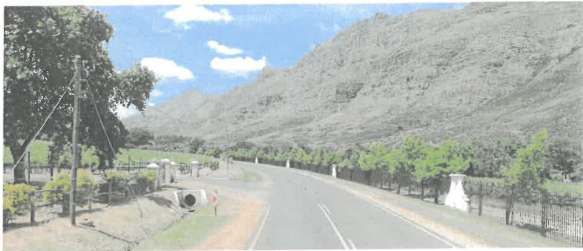
Image 1: The Jonkershoek Road runs perpendicular to the entrance of the proposed site property which is characterized by woodlands and winelands with a stormwater outlet next to the entrance point. Source: Google Earth Street View
