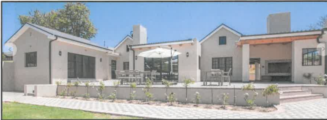
Figure 4: The main dwelling that will be converted into a tourist accommodation establishment with 5-rooms
