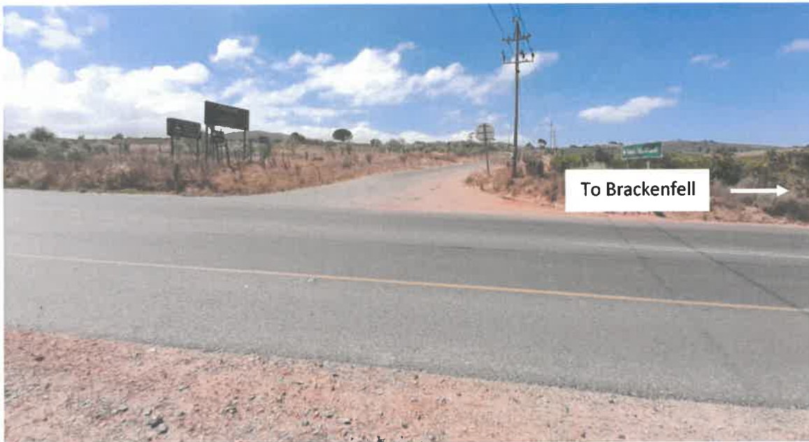
Figure 3: Photo of Bottelary Road/Fischers Road Access Point (looking down Fischers Road)
