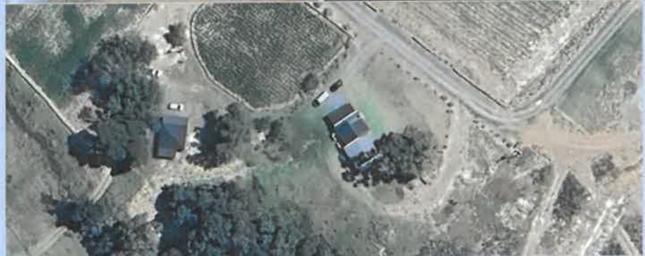
Existing employee house to be utilised as a tourist facility
