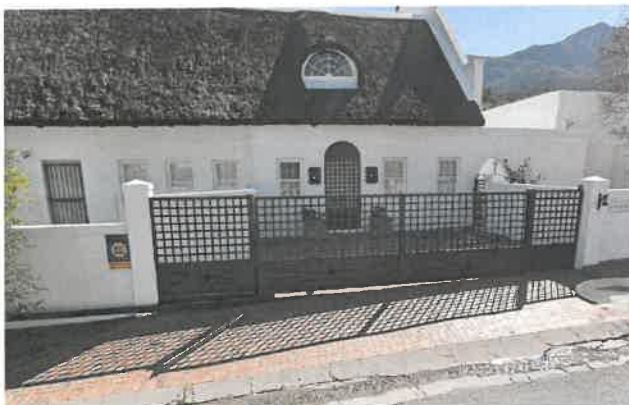
Figure 5: Parking on-site on Uitkyk Street side
