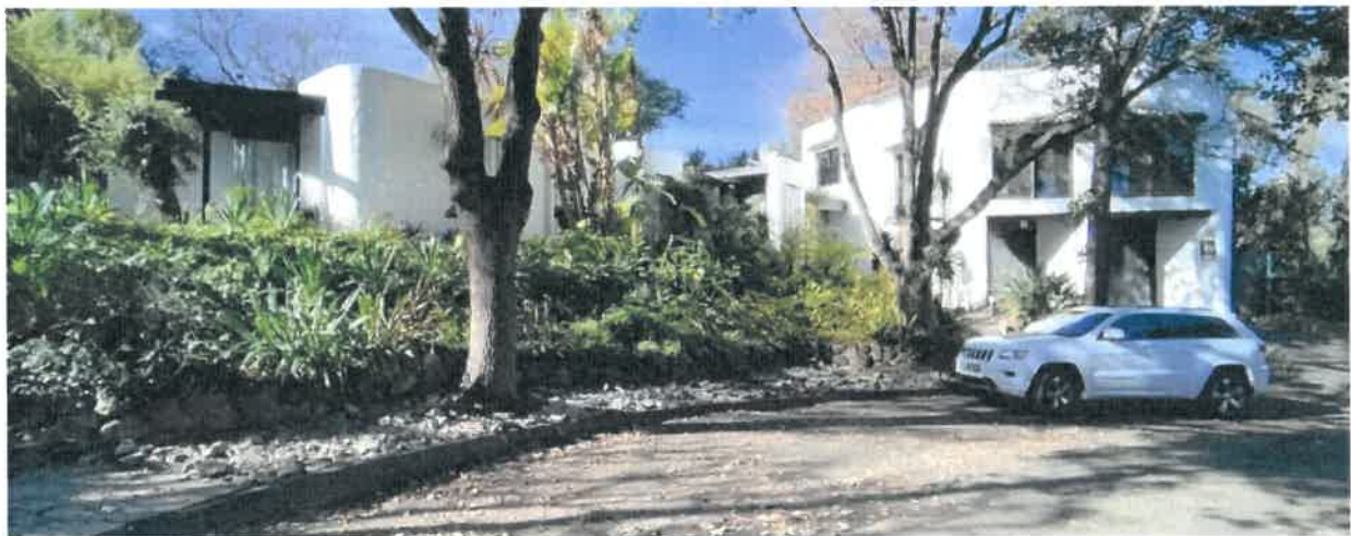
Figure 1: Street elevation of the dwelling on erf 5085, Stellenbosch.
