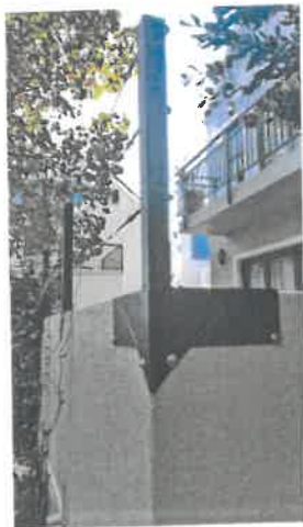
Fig 2. Steel and Wire Fence
