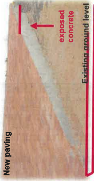
Figure 51: Haunching may not be exposed
