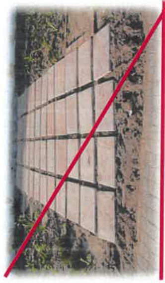
Figure 50: Pavers are not flush with road.
