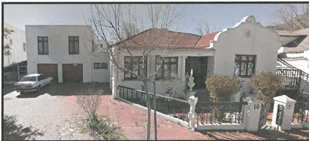
Figure 3: The existing dwelling on Erf 1150, Stellenbosch
