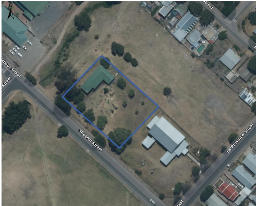
Fig 2. View of Property
