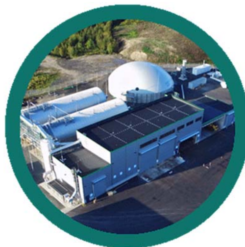
Figure : Biogas plant, Jönköping
