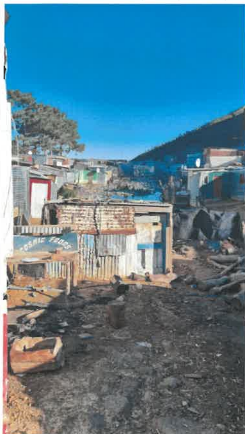
Figure 6: Some of the units located within the disaster area
