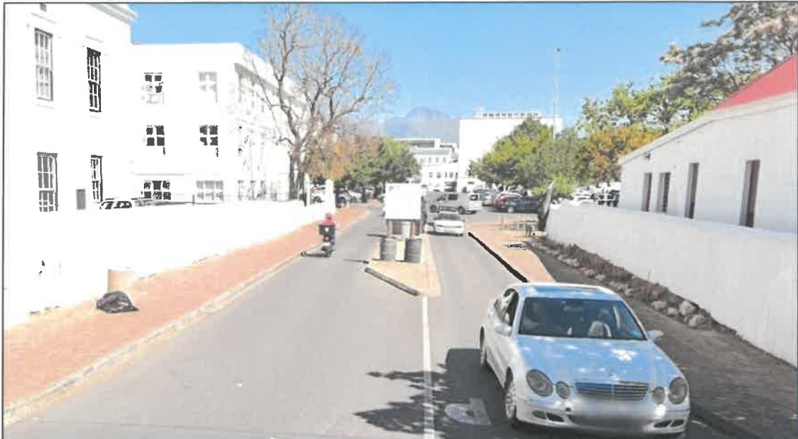
Figure 6-7: Victoria Street Access
