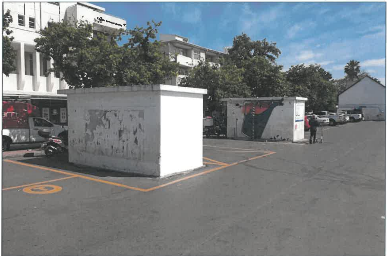
Figure 2-15: View of decommissioned public toilets on west side of the site (looking northwest).
