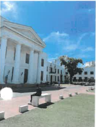
Figure 8D: View across the civic node facing Plein Street.
