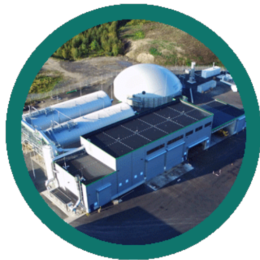
Figure : Biogas plant, Jönköping
