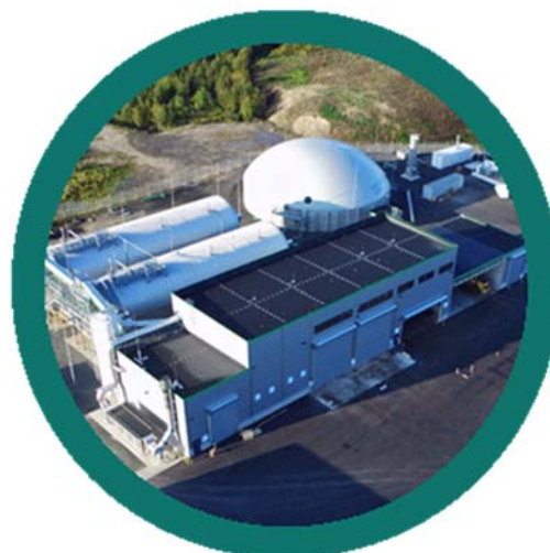
Figure : Biogas plant, Jönköping
