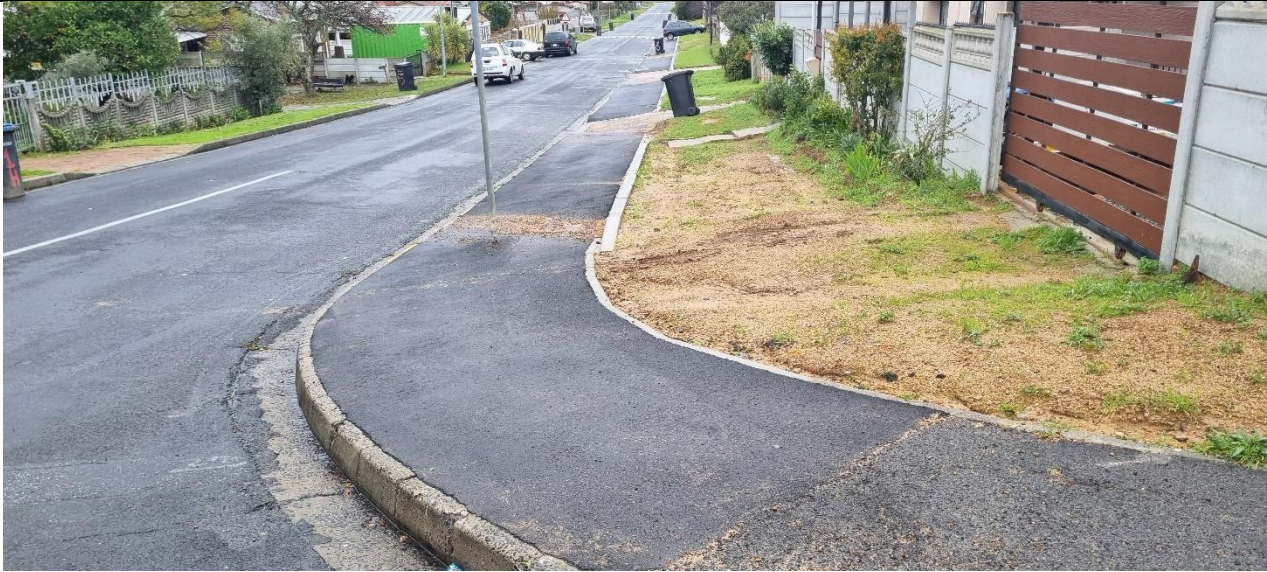
Site Photos (Hahn Street)
