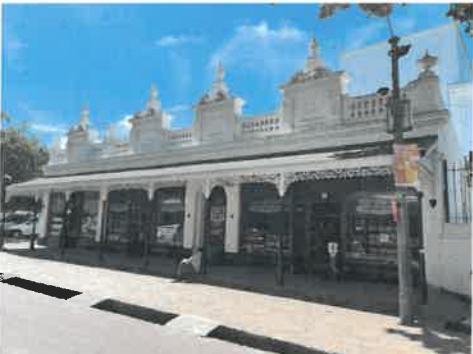
Figure 8J: Protected heritage building adjacent to the site along Andringa Street.
