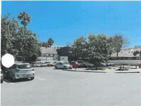
Figure 8G: View looking north-west to the backs of the heritage buildings at the corner of Andringa and Victoria Streets.
