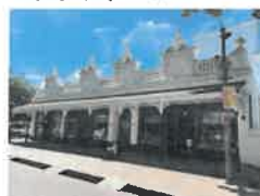
Protected heritage building adjacent to the site along Andringa Street.
