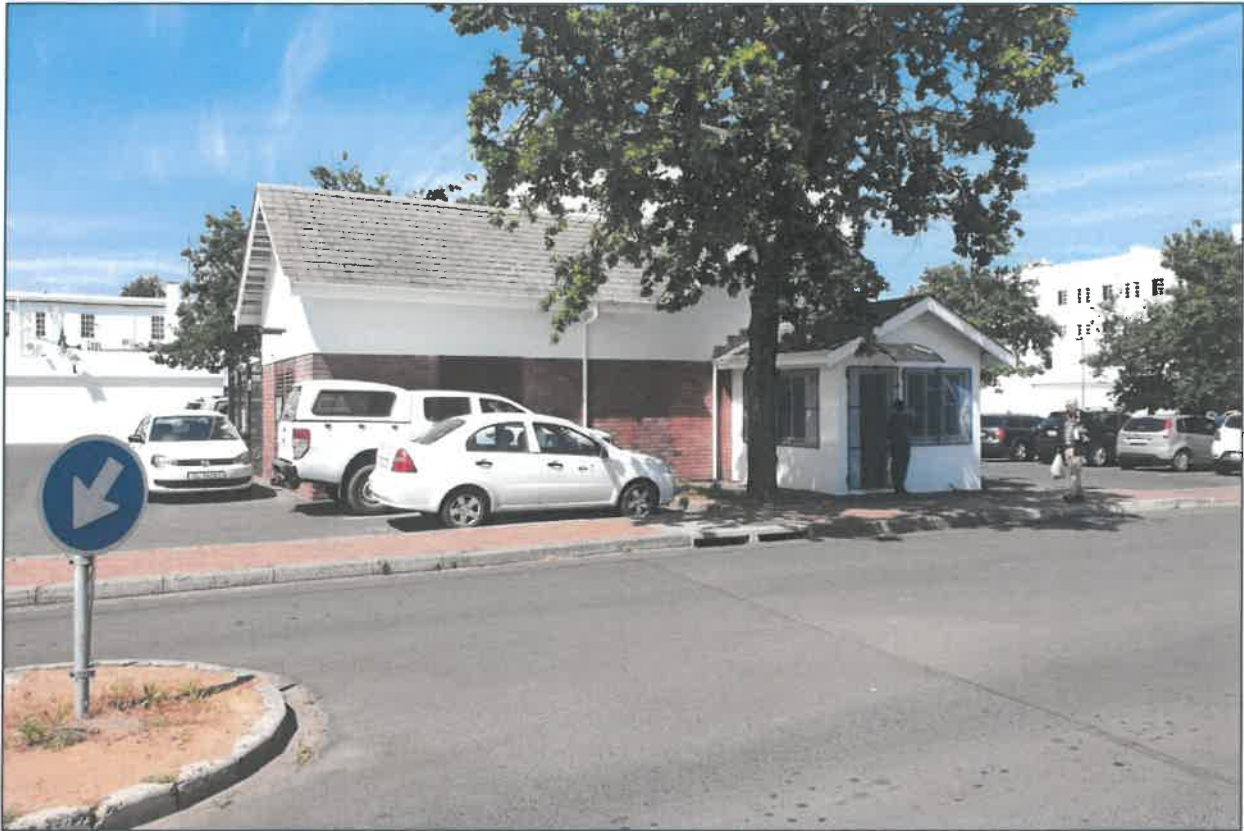
Figure 2-14: View of electrical substation from the parking lot (looking south-southwest).
