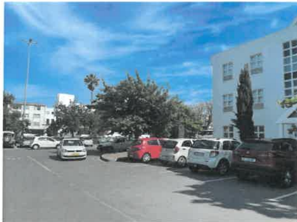
Figure 8C: View from the north-east corner of the parking lot, looking north-west.
