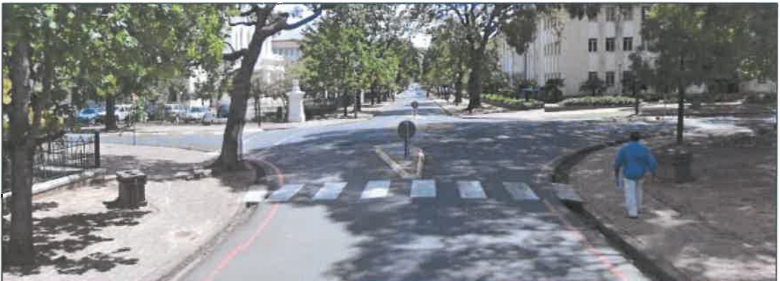
Figure 6-11: Pedestrian Crossing at the Victoria Street / Ryneveld Street intersection
