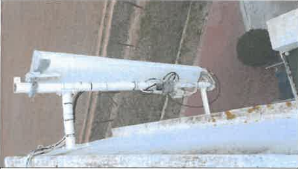
Sector 2 – Existing Antenna to be replaced with Hexaband and 5G antenna
