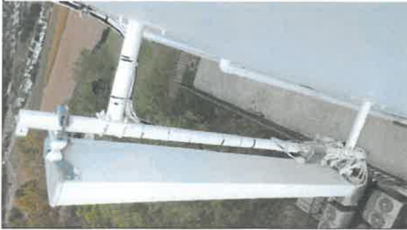
Sector 1 – Existing Antenna to be replaced with Hexaband and 5G antenna
