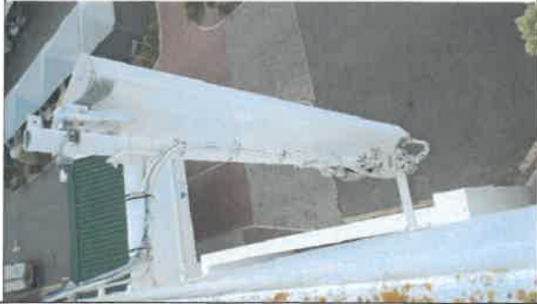
Sector 3 – Existing Antenna to be replaced with Hexaband and 5G antenna
