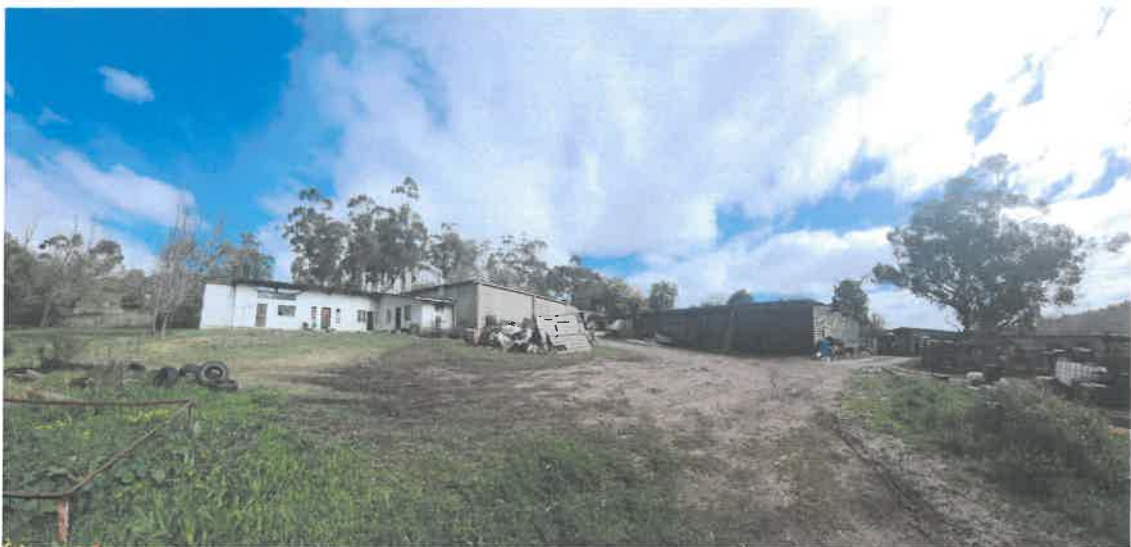
Figure 1: Buildings, structures and implements scattered across the property.
