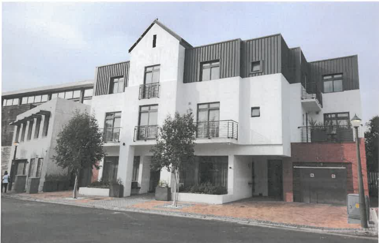
Figure 1: Street façade of Hotel Krige.
