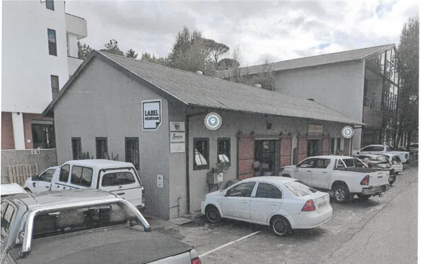
Figure 3: Façade and Parking of Erf 14165, Stellenbosch
