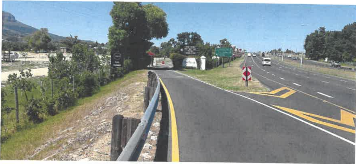
Slip off lane along the R44 Main Road
