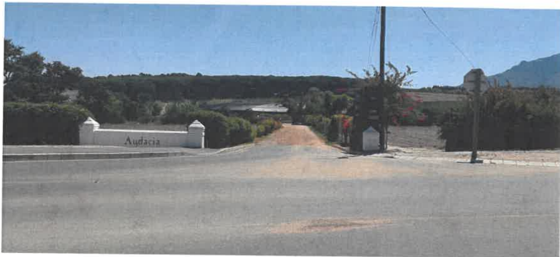
Upgraded access road off the Annandale Road.
