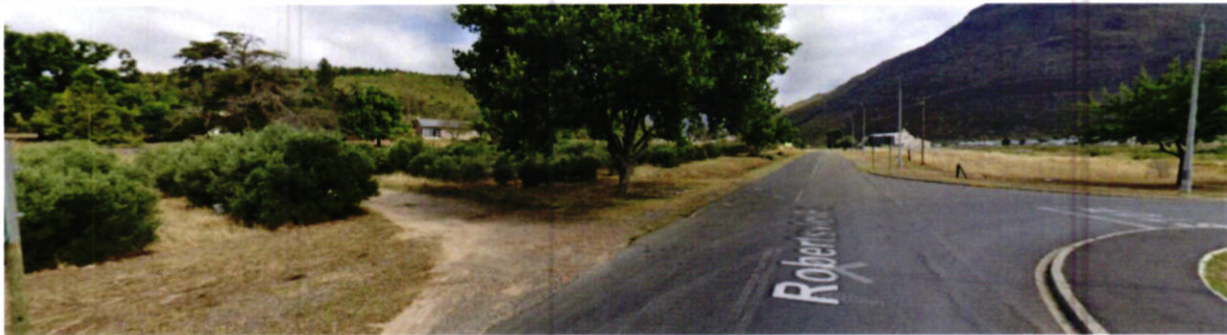
Image 2: Street view south from Robertsvlei Road showing the intersection with Bergendal Street on the right and existing access to the municipal houses visible on the left. This is also the proposed new entrance to the school. (Source: Google Earth)
