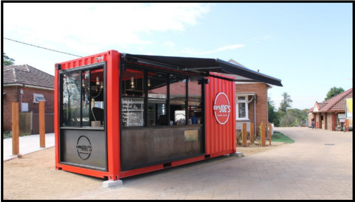
Figure 4: An example of a removable container that has been converted into a stall
