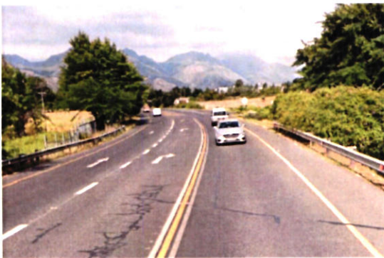
Photo 1 MR191 Eastbound View towards the Farm Access
