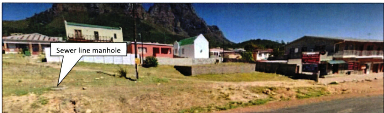
Photo 2: View of the property from the R310 with the slab, manhole and electrical infrastructure clearly visible.
