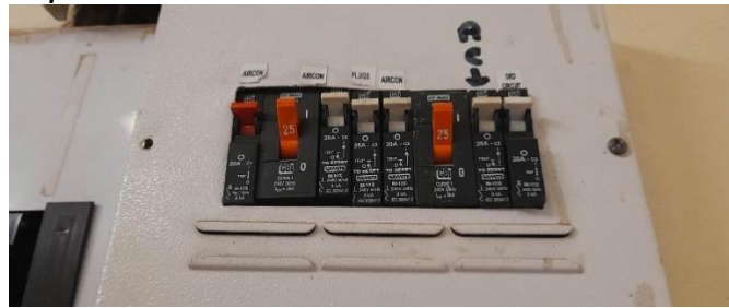
Figure 4 Main DB Expansion circuit breakers
