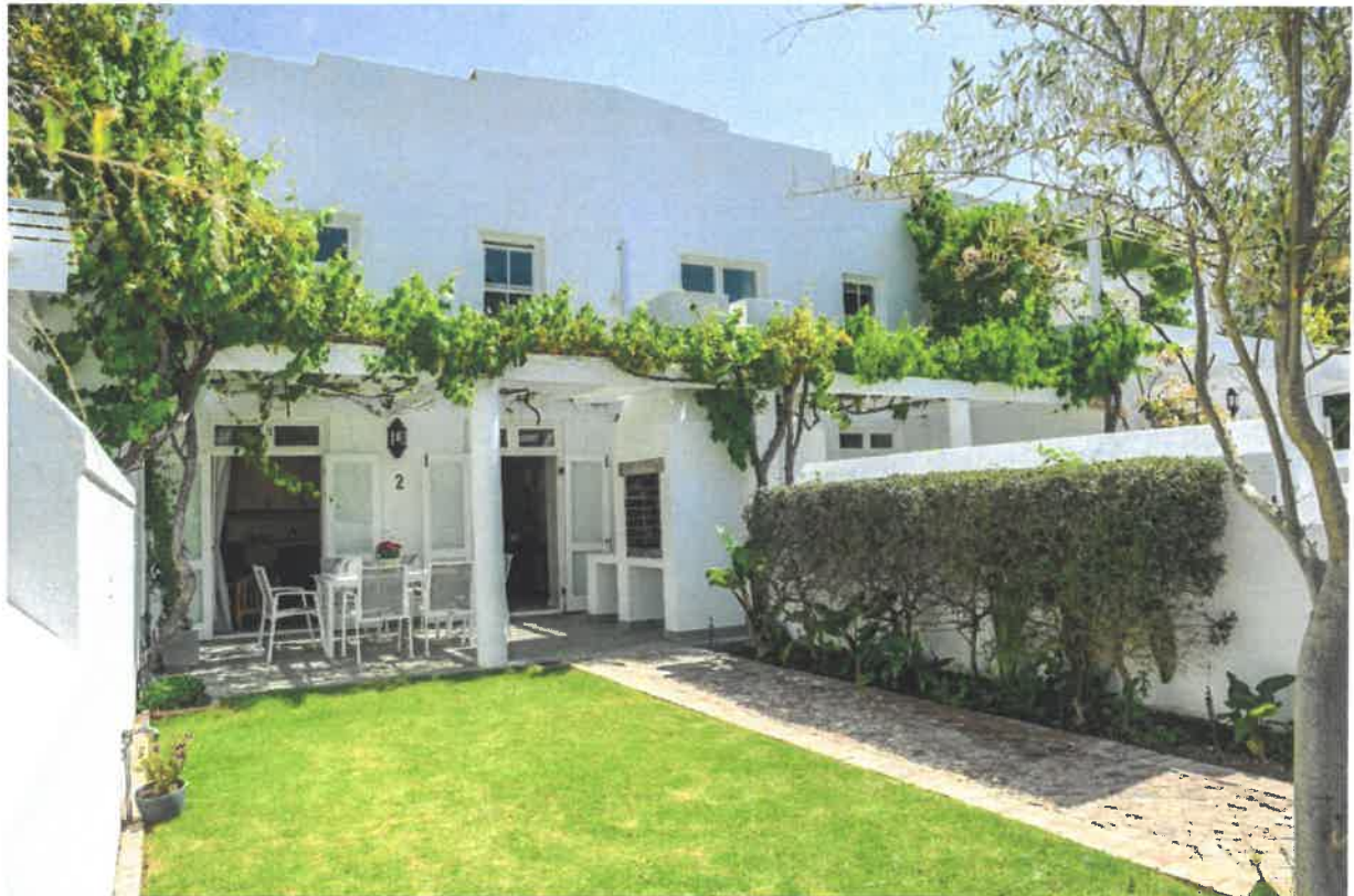
Figure 12 Existing four 2-storey cottages
