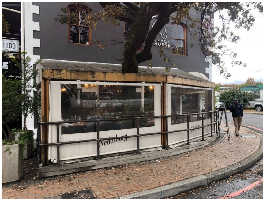
Fig 3. Current area being used for outdoor dining
