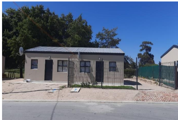
Longlands Housing Project
