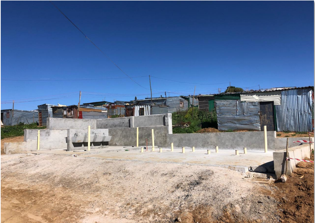
Figure 37: Construction of basic services, Watergang Informal Settlement
