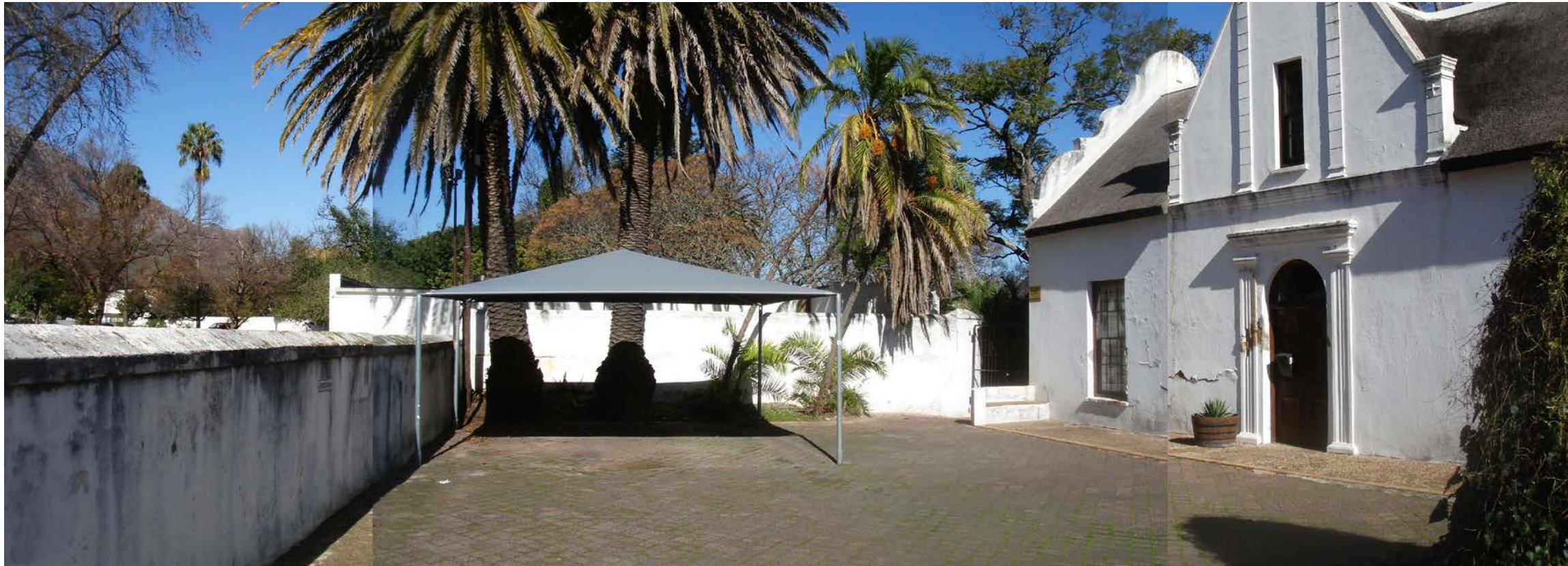
Figure 18: View of Leipoldt Court looking south.
