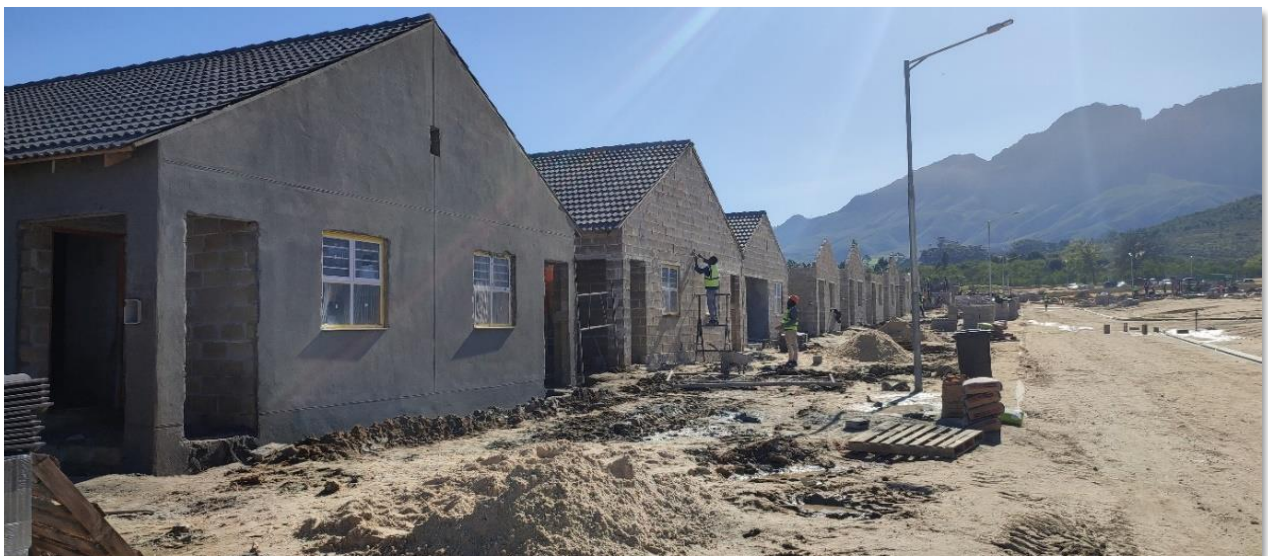
Figure 38: Ida's Valley Housing Development Project
