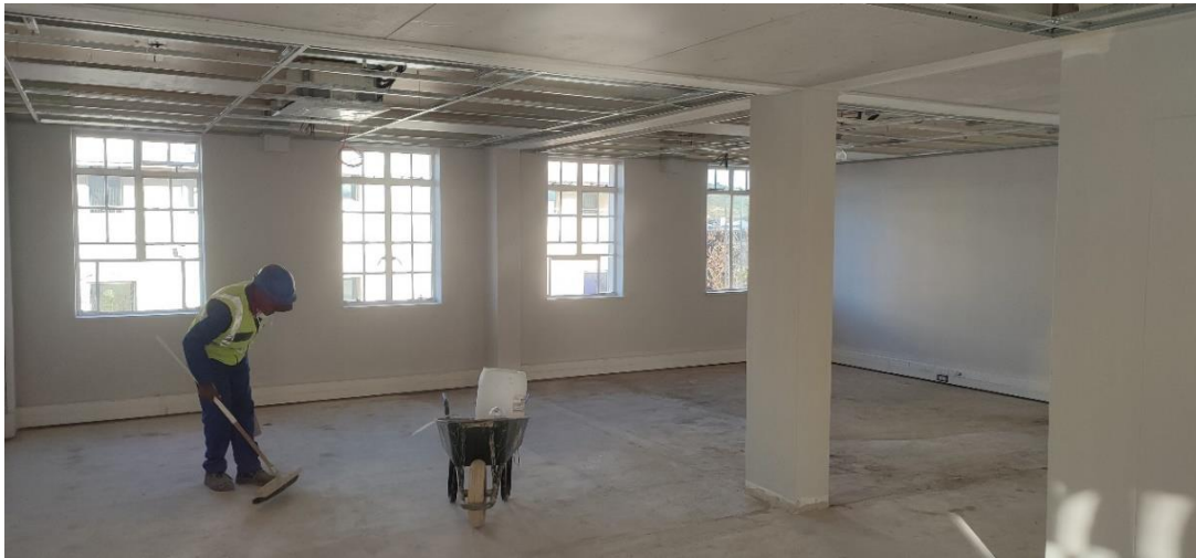
Figure 41: Upgrading of the NPK Building
