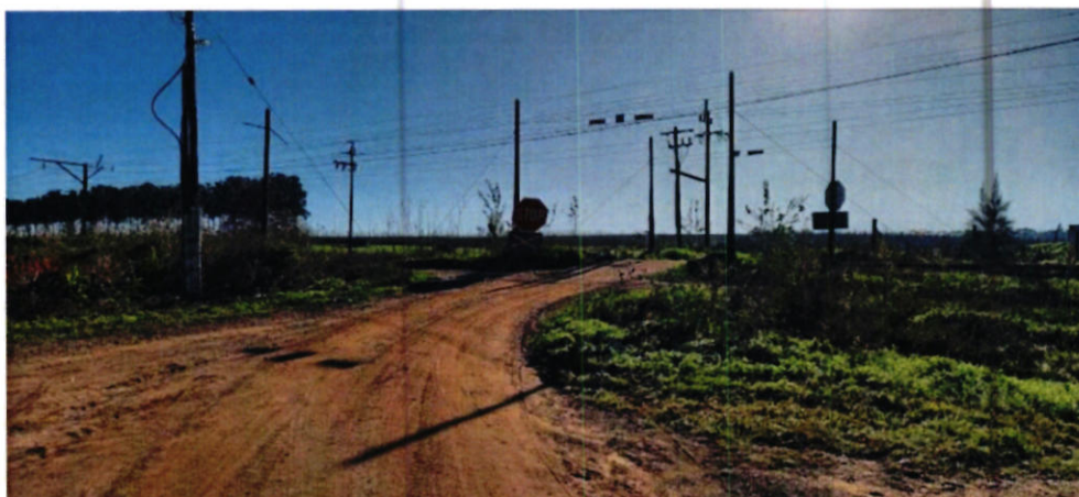
North view of the railway line bordering the subject property
