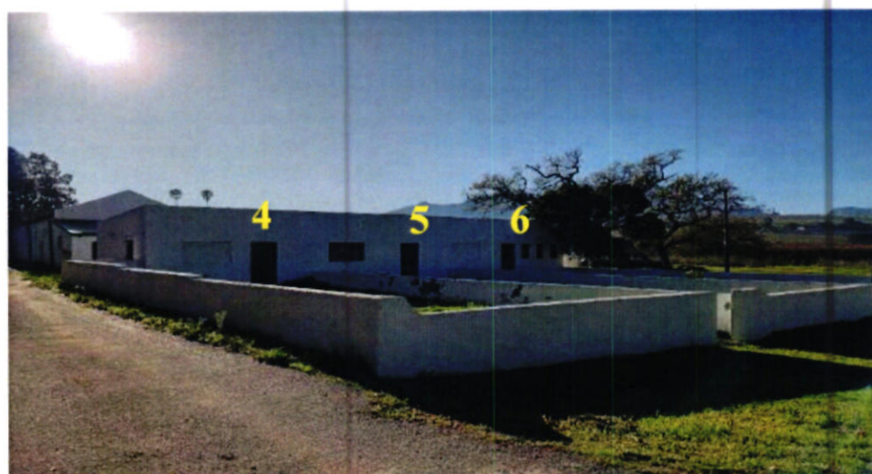
Vacant employee houses to the north of the existing cottage
