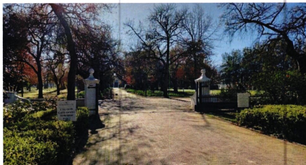
Entrance to the subject property from the R304
