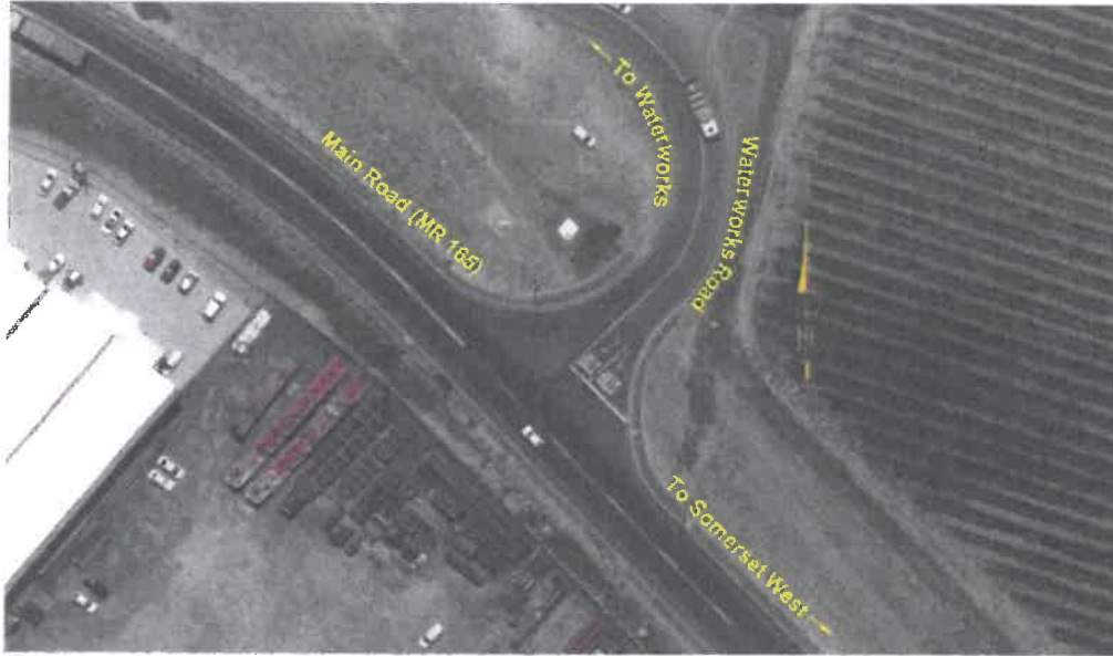
Photo 4 : Existing Main Road/Waterworks Road intersection lane layout
