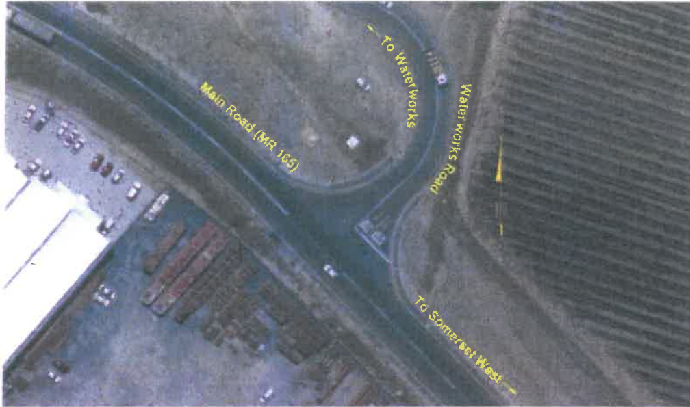
Photo 4 : Existing Main Road/Waterworks Road intersection lane layout
