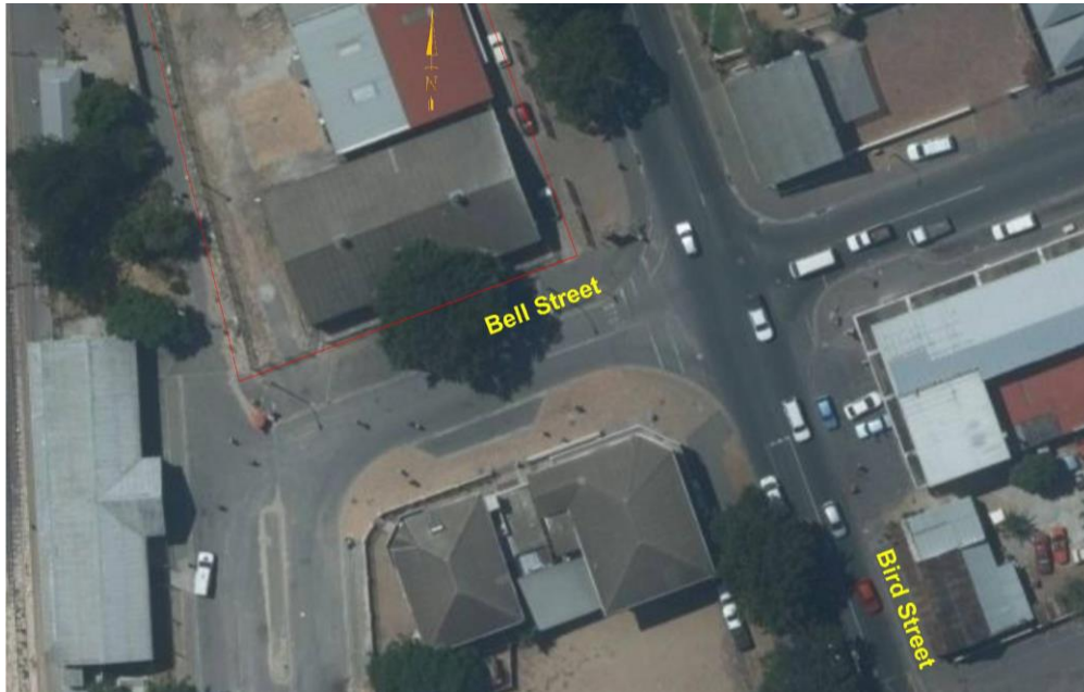
Photo 2 : Existing Bird Street/Bell Street intersection lane layout
