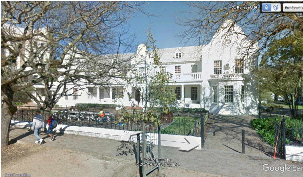
Fig 5: Streetview of Neethlingshuis offices
