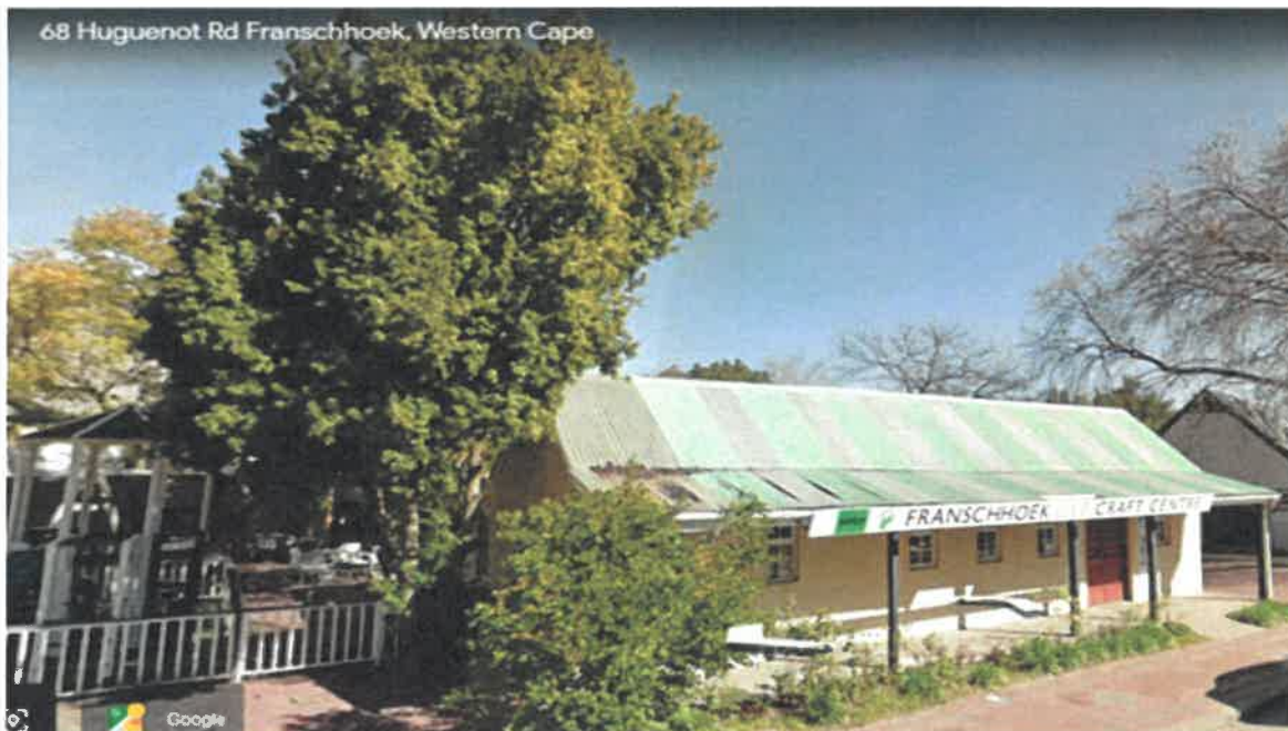
Streetview of building
