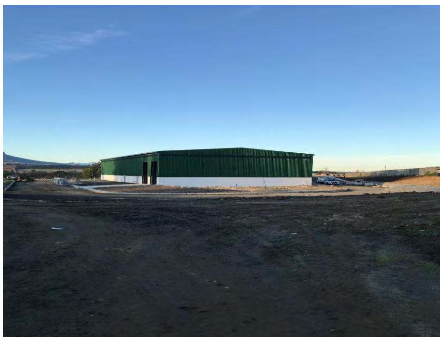
New MRF building under construction
