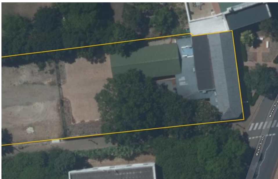
Figure 2: Aerial view of site showing the existing structures on site.
