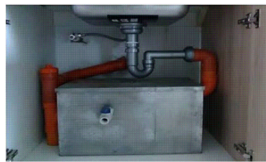
UNDER COUNTER GREASE TRAP
